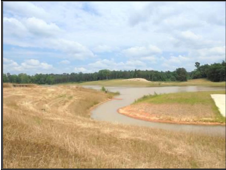
Viewing spillway in the northwestern area of lake
