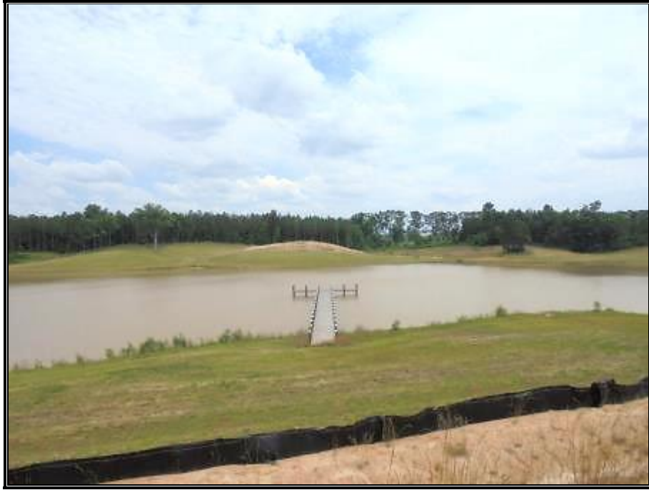
Viewing south across lake and pier
