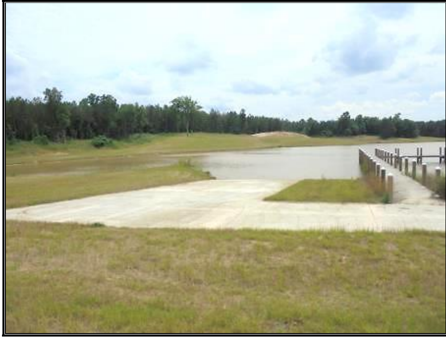
Viewing boat ramp in the northeastern portion of lake
