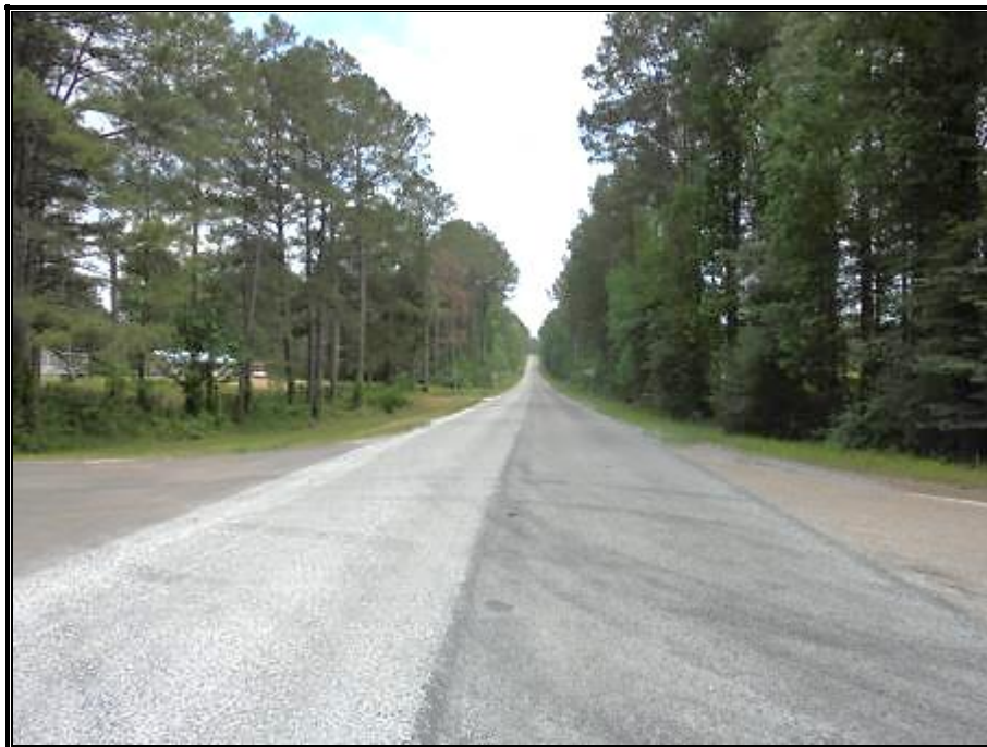
Viewing south along Hwy 17 in front of subject property
