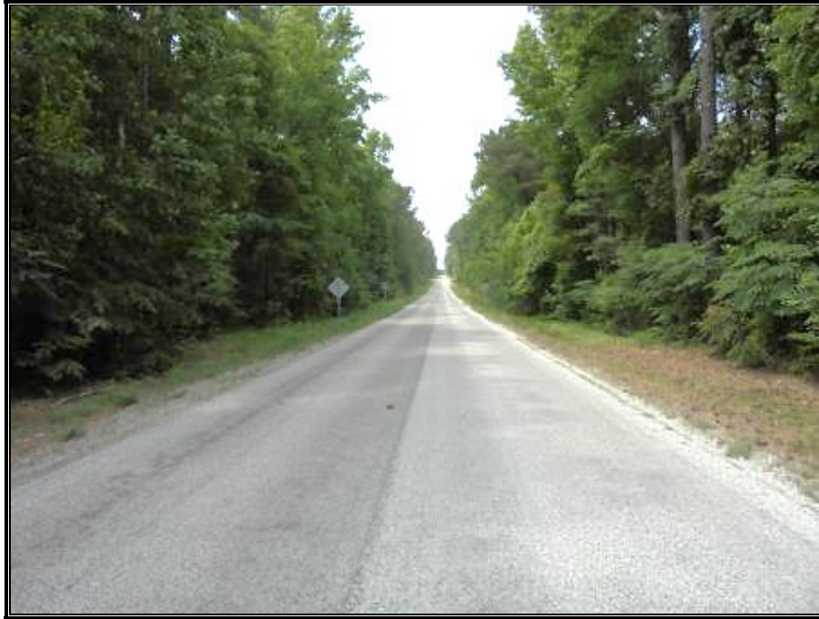
Viewing north along Hwy 17 in front of subject property
